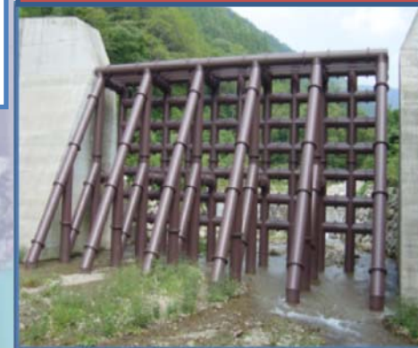
Steel pipe SABO dam as downstream
