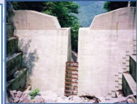
Concrete slit SABO dam and steel bars
