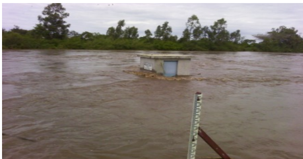
Automated River Gauging Station
