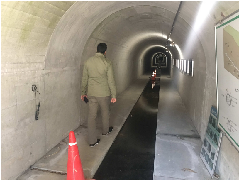
Figure 4.20: Ground Water Drainage Works In the Kamenose area.
