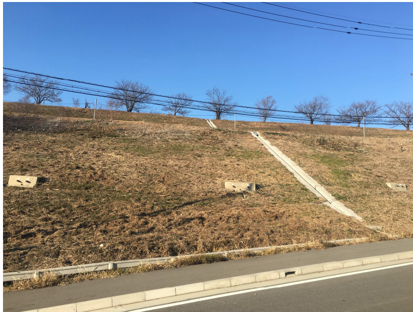
Figure 4.21: Surface water drains and Anchors
