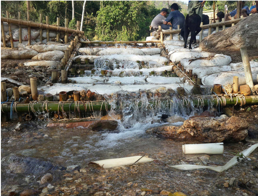
Figure 4.31 check dam for water retention in Thailand
