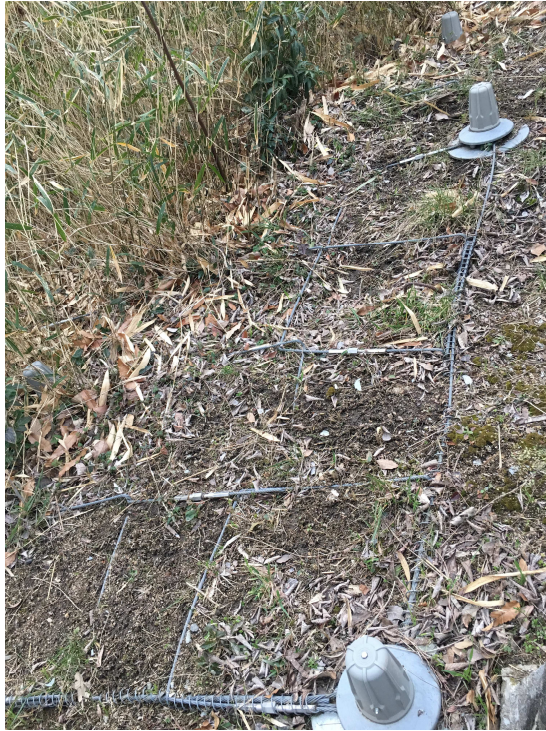
Figure 4.23: nailing network system in Kobe University.
