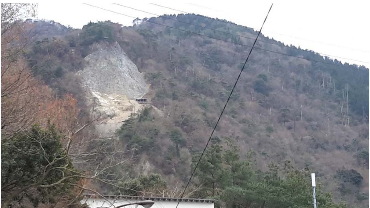
Landslide near Arima Onsen, Hyogo
