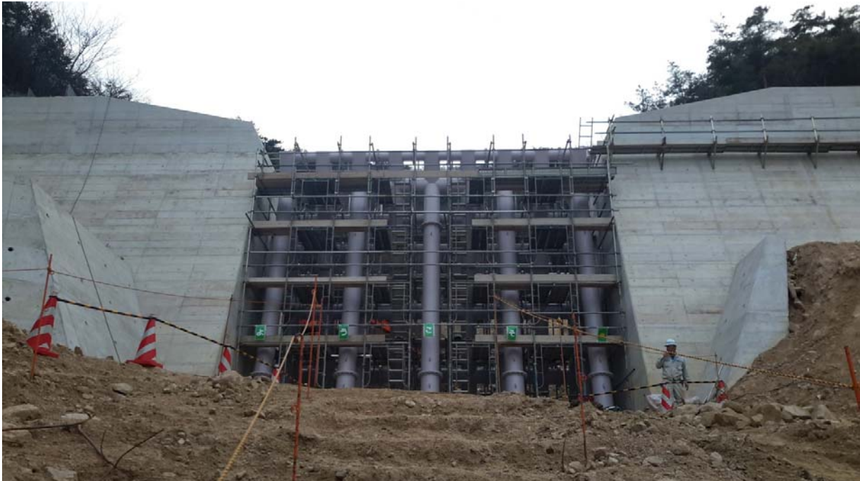
Steel grid Sabo Dam at Mt. Rokko
