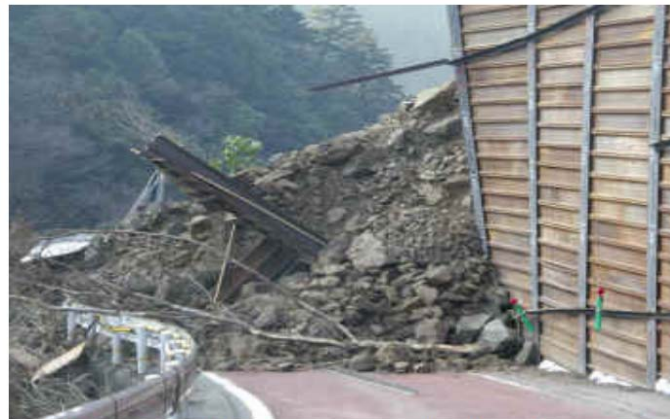
Damaged temporary protection fence
