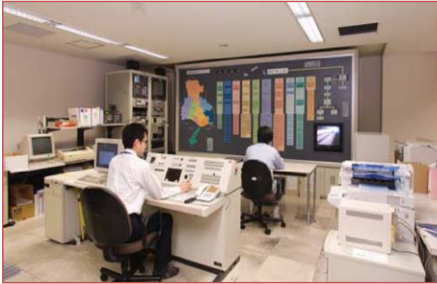
Figure (16) Network Control Room
