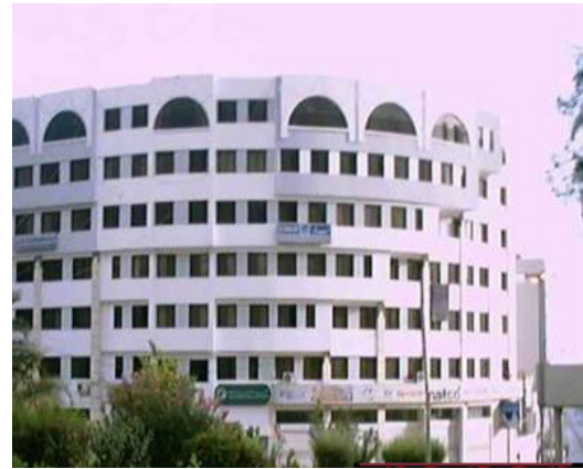
Figure.(9) RM structure , RC filled with stone
