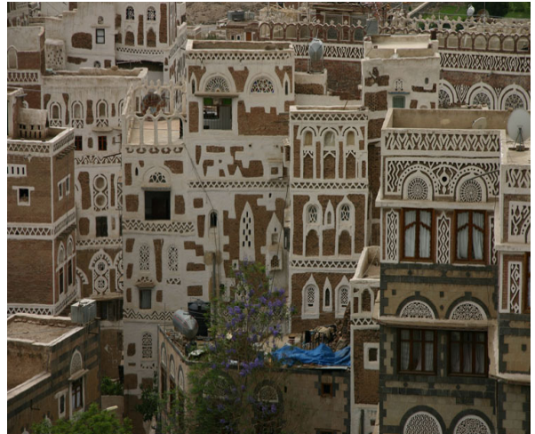
Figure.(7) URM Masonry Building (Brick ,stone and clay
