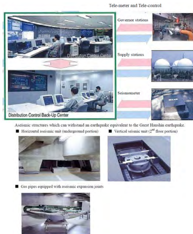
Figure 37. Seismic resilience measures by Osaka Gas Engineering
