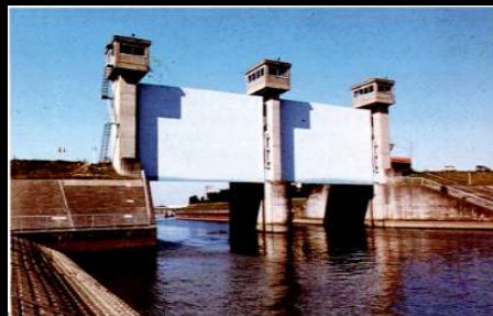
Gate to protect river water to use during drought
