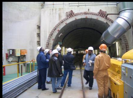
Installation of underground river pipe
