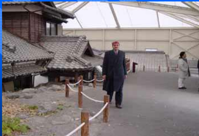
Damaged Houses due to Volcanic activities- Nagasaki
