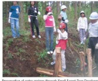
Preservation of water springs through Small Forest Dam Development
